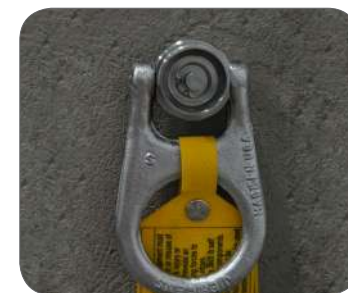
Figure 2: Example of a cast-in eyebolt anchor.
