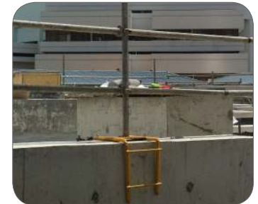
Figure 31: Example of parapet edge protection design.
