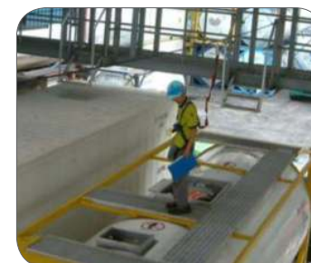
Figure 36: Drive-in anchorage and lifeline structural system.
